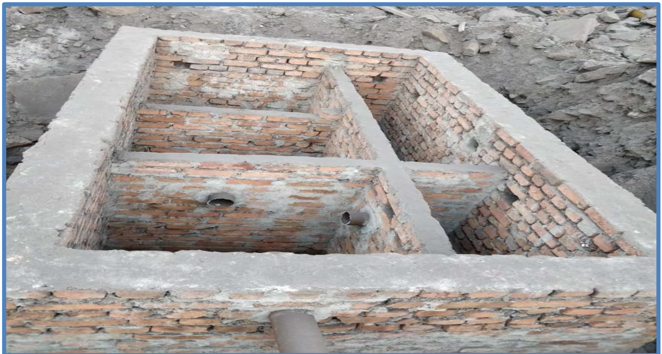
Picture 10 – Oil & Grease Trap
