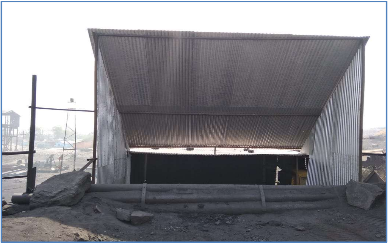
Picture 7 – Enclosed Coal Handling Plant
