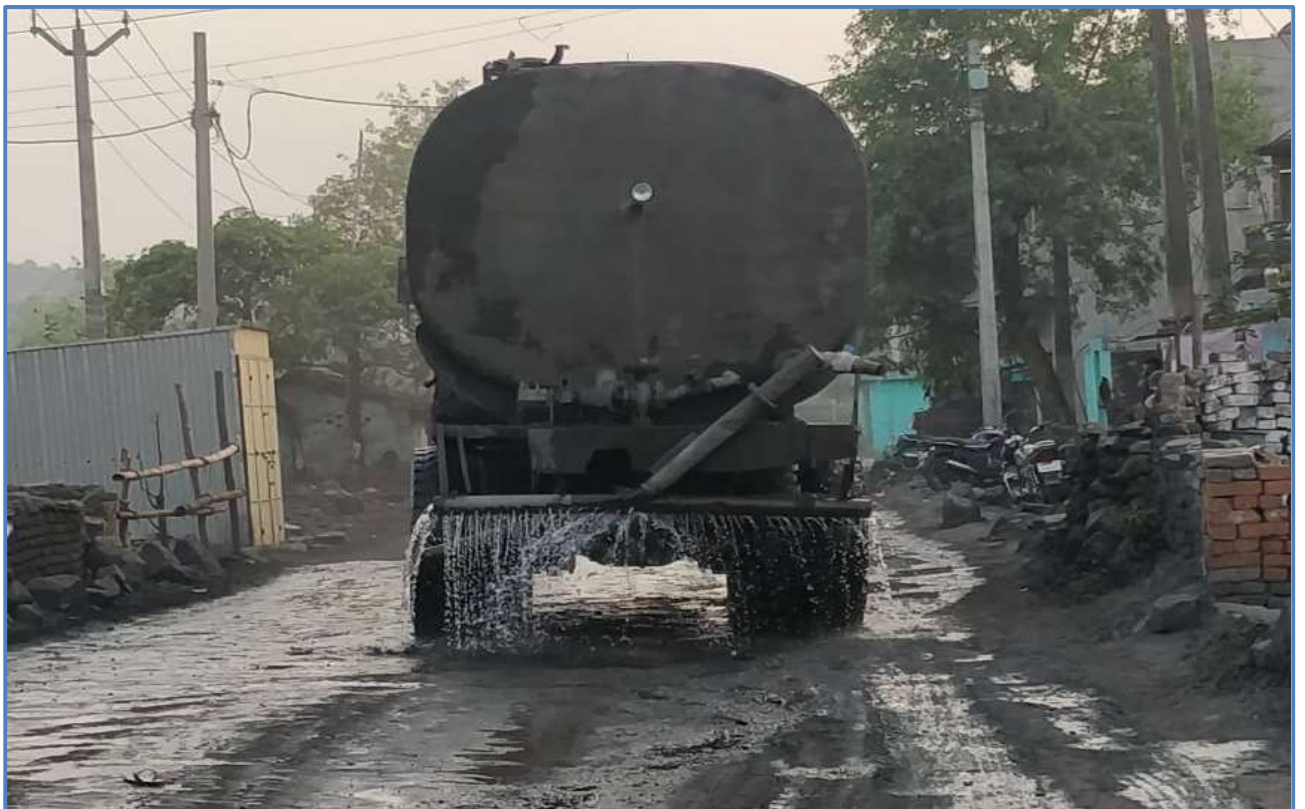
Picture 2 – Water Sprinkling on Transportation Road
