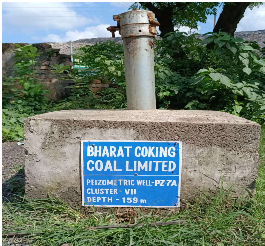
Picture 12 – Piezometer well
